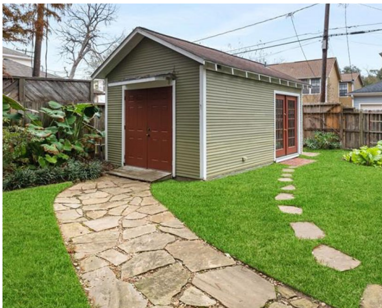
Figure 2- existing garage to be demolished
